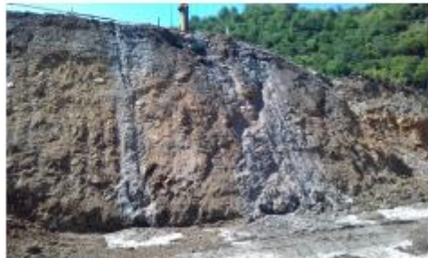
Photo 3. Interchange 202. Non-Conformance: Concrete washout on the ground. Misc. truck drivers should be informed about that washing out of Concrete. Chemicals is allowed only in Washout pits. If it is necessary, additional washout pits should be made.
