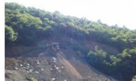
Photo 5. Tunnel 03, Portal Non-Conformance: While excavation and drilling of tunnel portal, spoiled soil and rocks are falling in to the River. Bottoms. All disposed material should be removed and river bank protection should be made.
