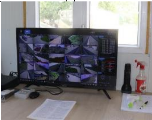
Photo45: Control Room of CCTV Cameras
