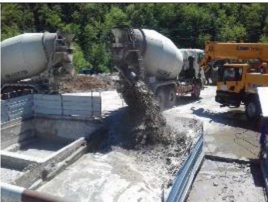
Photo39: Concrete Mixer Washout Pit
