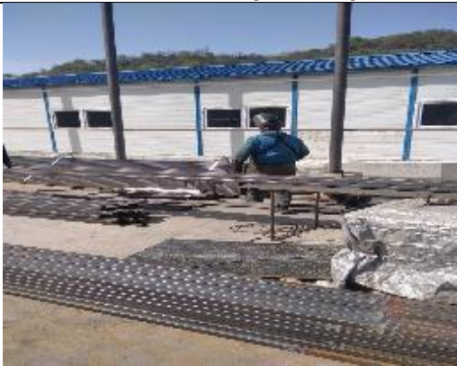
Photo43: Welder using Protective Equipment
