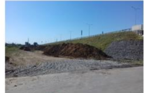
Photo 8. Interchange #4 AT Good Observations: Topsoil storage in progress. When accumulation of topsoil will be completed it must be fenced with geotextile and drainage channel should be made, to avoid erosion and washout.
