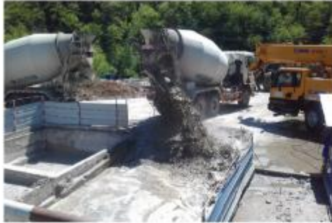
Photo 6. Interchange N11 Good Observation: Washout concrete mixer truck in to proper washout pit.
