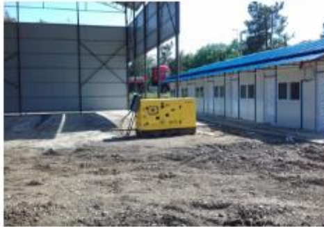
Photo 1. Interchange #00: Noe Conformance Diesel Generator is placed on the Ground without Drip tray (Drip trays are ordered and will be presented as soon as possible)
