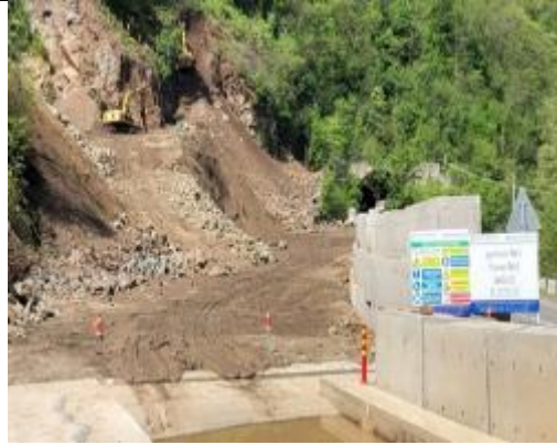
Photo18: Site Name Indicative and Construction Site Safety Signs
