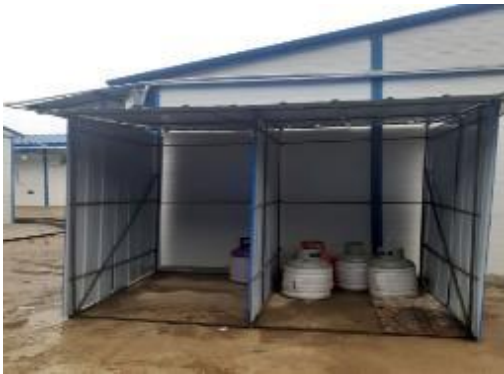
Photo35: Gas Cylinders inside the Shelter
