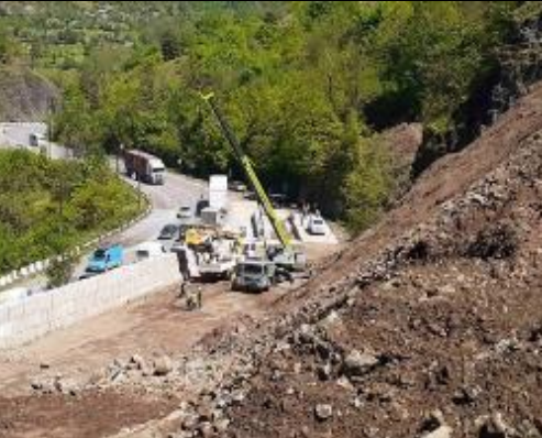
Photo13: Preparatory Work for Tunnel
