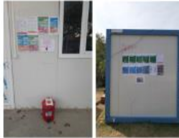
Display of publicity brochures in the construction site accommodation area
