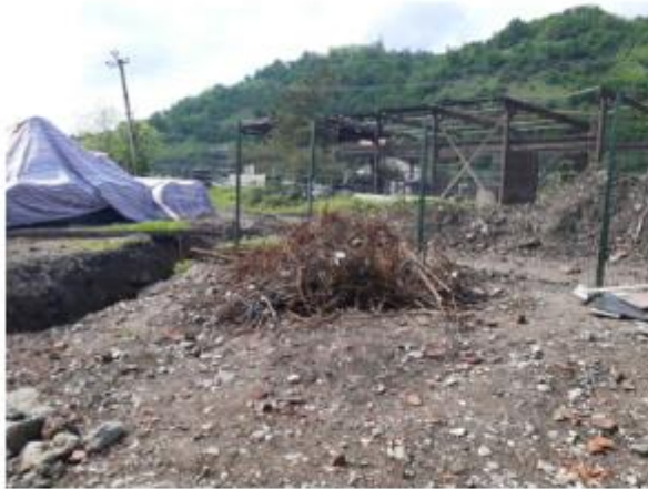
Photo 3. Interchange #22: Non-Conformance: Metal waste collecting/storing area must be fenced;
