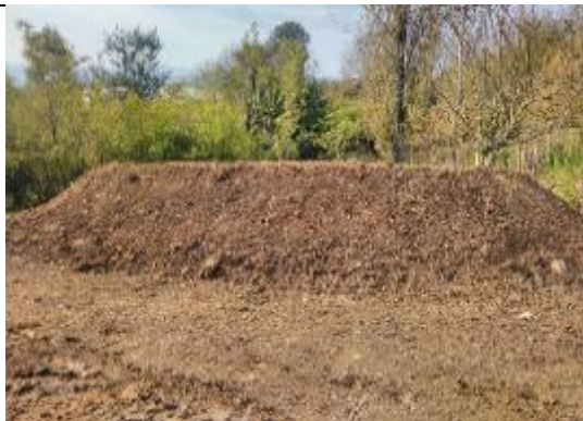
Photo47: Topsoil Storage at Access Road 2
