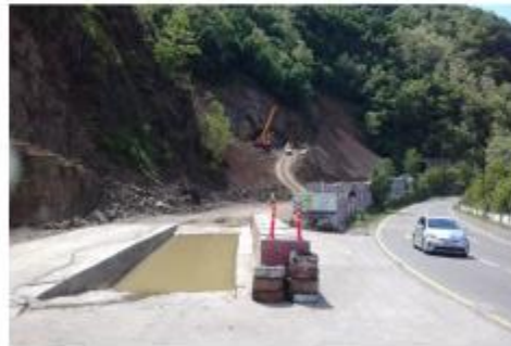
Photo 7. Interchange N11, Tunnel #2 Good Observations: Washout for tires of trucks are available on most of the sites.
