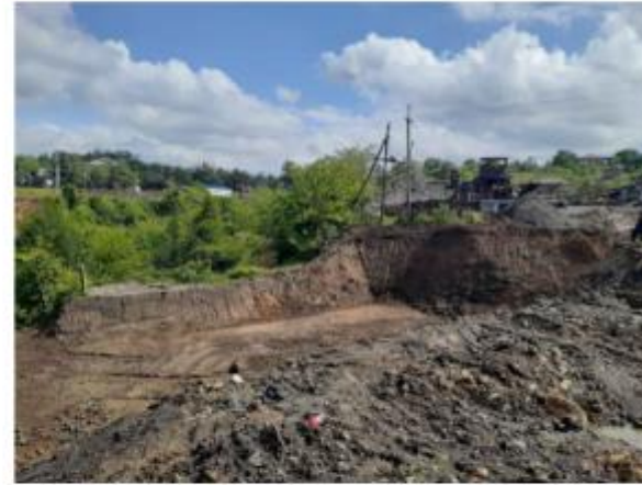
Photo 4. Interchange #22: Non-Conformance: The excavation area must be fenced with protective guardrail;
