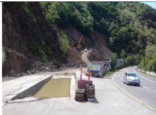
Photo40: Washout Pits for Tires
