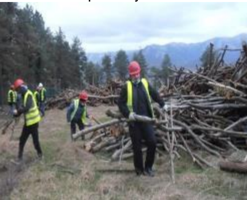
Photo15: Tree Cutters and Designated Storage Area
