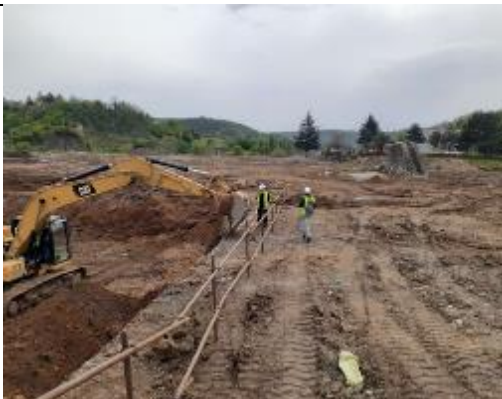
Photo16: Protective Guardrails in the Excavation Area
