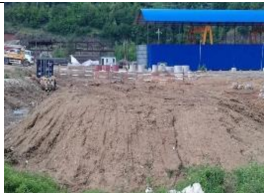
Photo48: Topsoil in Temporary Area
